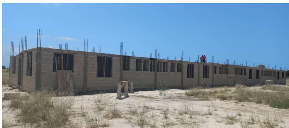
Construction of 12 Unit Hostel (Ground Floor) with ancillary facilities
