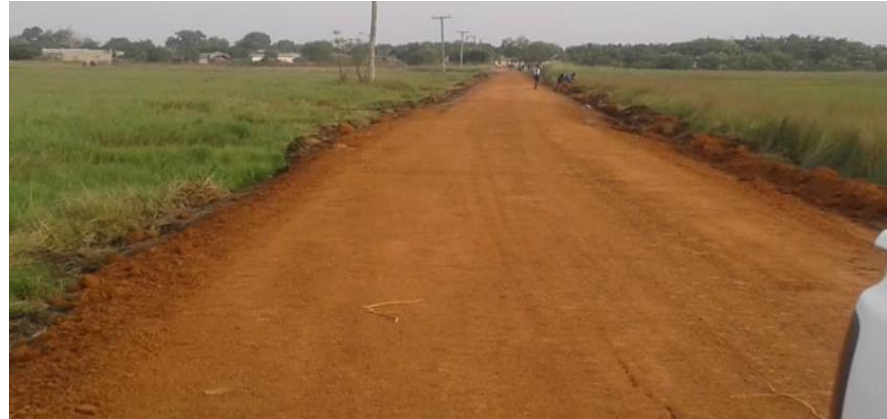
Reshaping and gravelling of road at Atiavi to Glime and Keta-Rose Pavilion road
