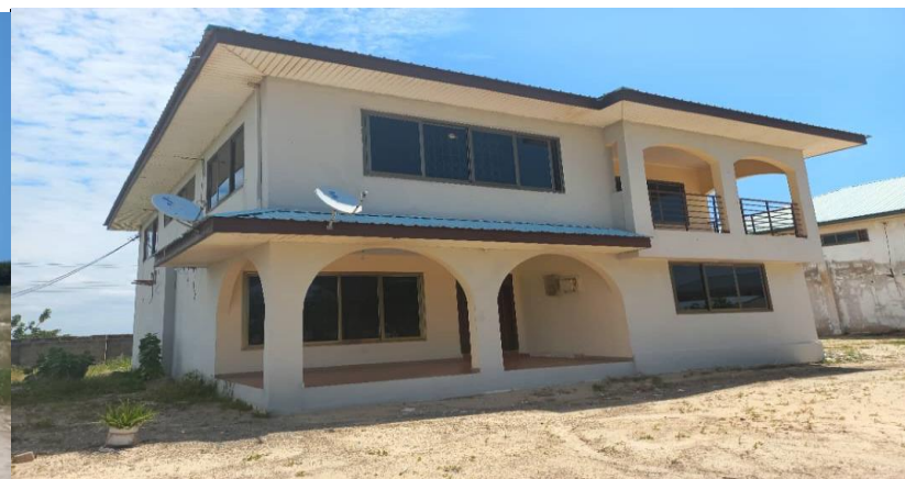
Renovation of Doctors Flat at Keta
