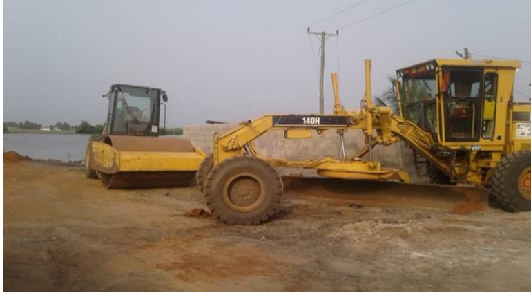
Reshaping and gravelling of road at Atiavi to Glime and Keta-Rose Pavilion road
