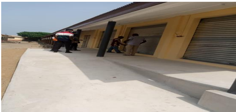
Construction of Lockable stores @ Keta
