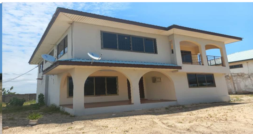
Renovation of Doctors Flat at Keta
