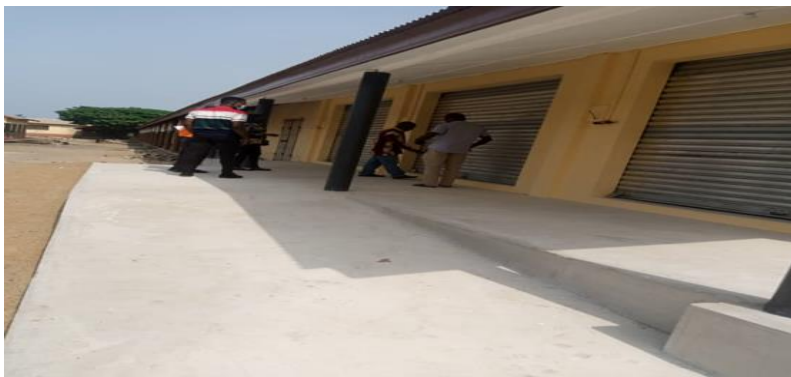
Construction of Lockable stores @ Keta
