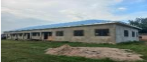
Construction of 3-Unit Classroom Block with ancillary facilities at Abor
